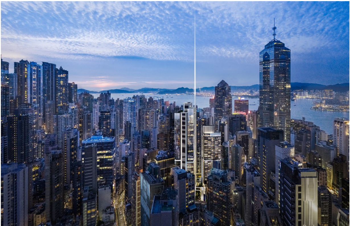
Central Crossing, slated for completion in mid-2026, has completed its topping out. Image credit: Central Crossing
